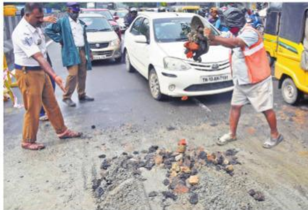
A pothole on the Poonamallee High Road at Kilpauk being filled with gravel and cement, in Chennai on Wednesday | R SATISH BABU
